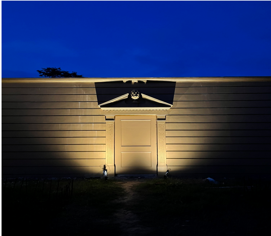
Staff Quarters Entrance — Same Standard, Every Corner
